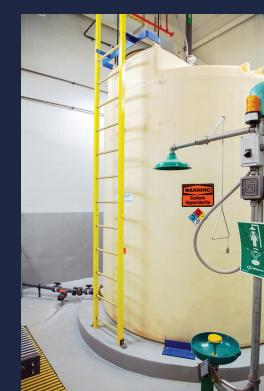
This tank of sodium hypochlorite, located in the CEPT Building, is used with both disinfection and odor control.
