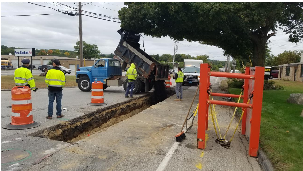
Figure 3 - Airport Road Sewer Work – Trench Box on right
