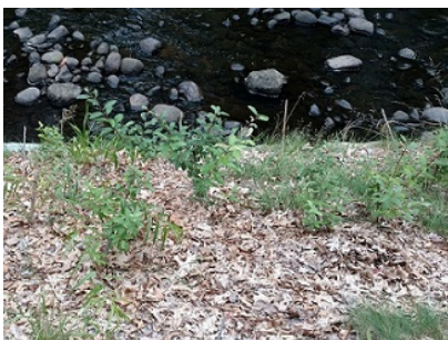
View of Stake Plantings in the Slope (Mixture of Black & Purple Willow Species) Showing Growth, After Installed as Dormant, Live Rooted Woody Cuttings.
