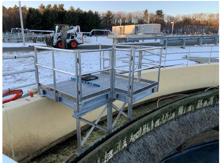
Figure 5 - 2nd Stage Clarifier Platform
