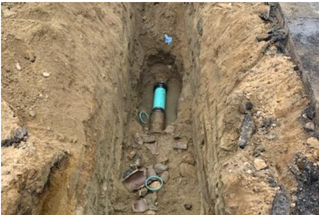
Photo 5: Spot Sewer Repair (Trench View).
