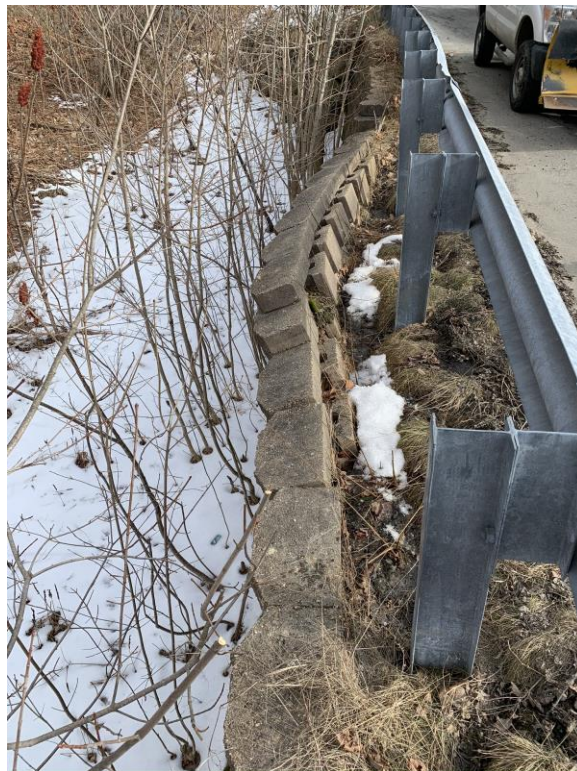
Figure 4 - Arn How Farm MSE Wall Failure
