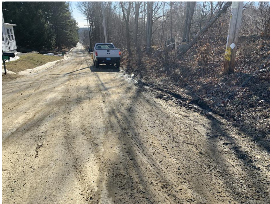
Figure 3 - Paved roadway covered in sediment from construction site
