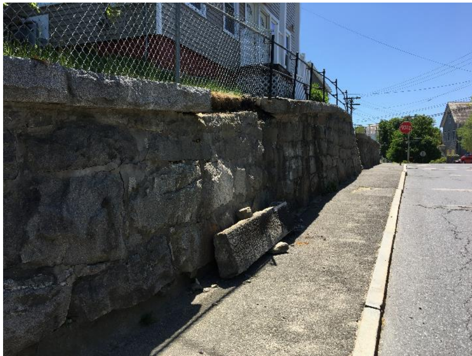
Figure 3 - Collapsing Wall
