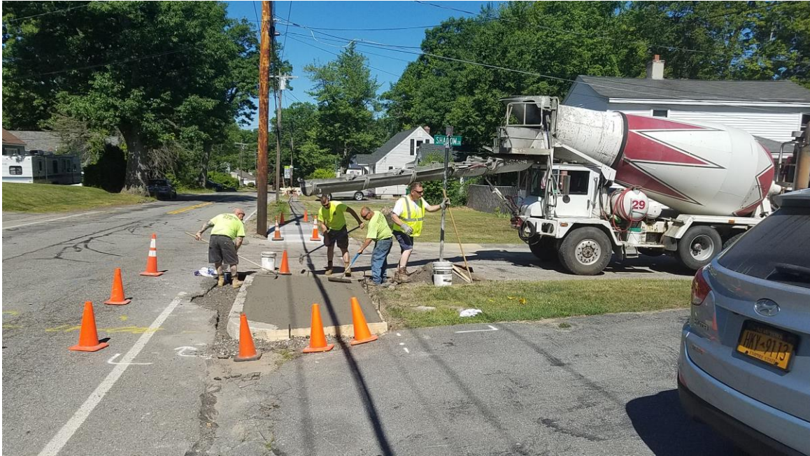
Figure 2 - Pouring of ADA ramps at Shadow Drive
