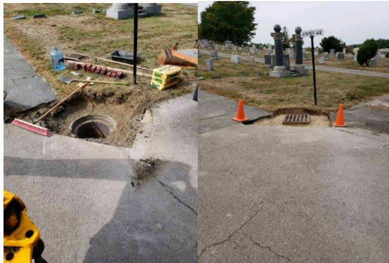
Figure 3 - Catch Basin Repair at Cemetery
