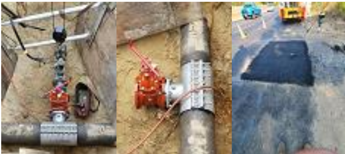
Figure 4- 8-in Water line insertion
