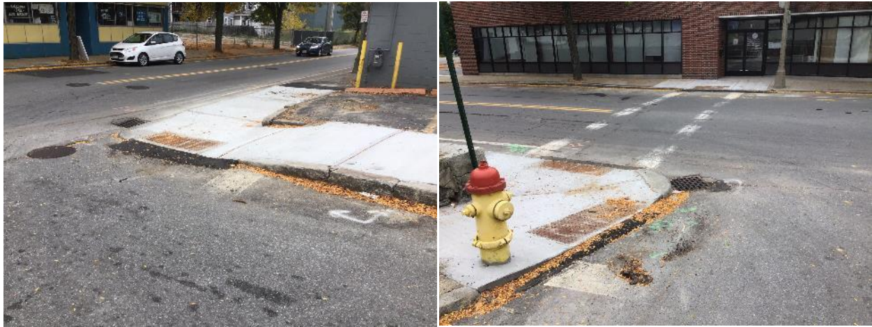
Figure 2 - ADA Ramps completed across Granite and Water Street
