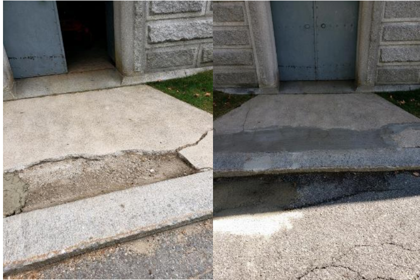
Figure 3 - Mausoleum Step Repair - before and after
