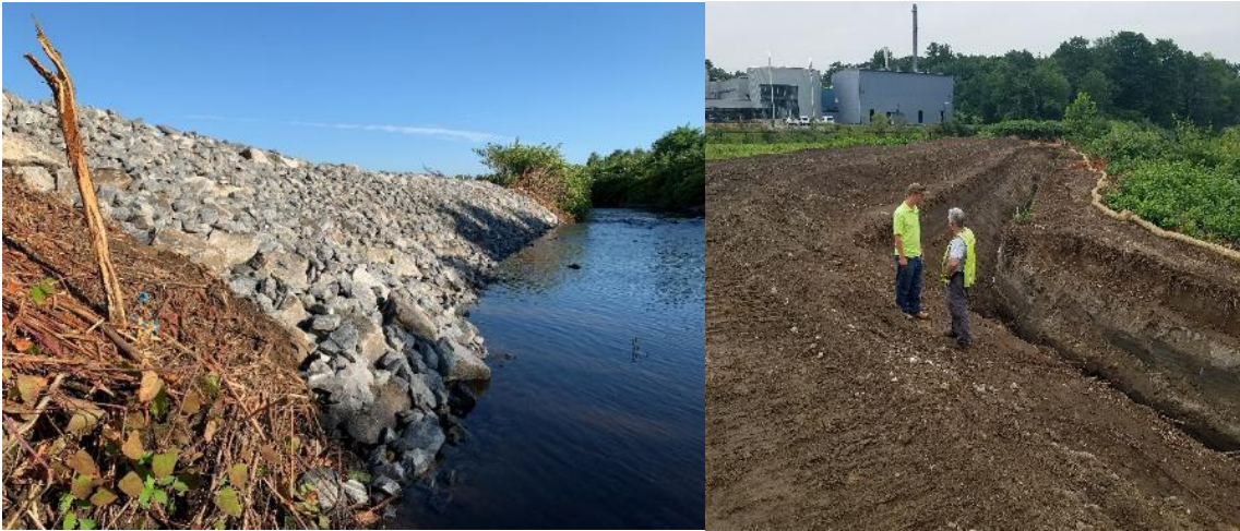
Figure 5: Erosion Stabilized River Bank (Nashua River, at the East WWTF).
