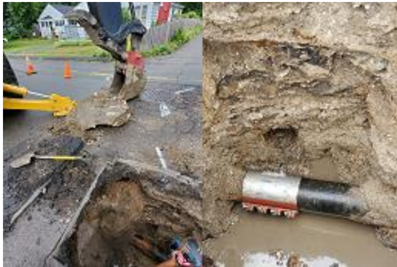
Figure 7 - Water Main break and repair
