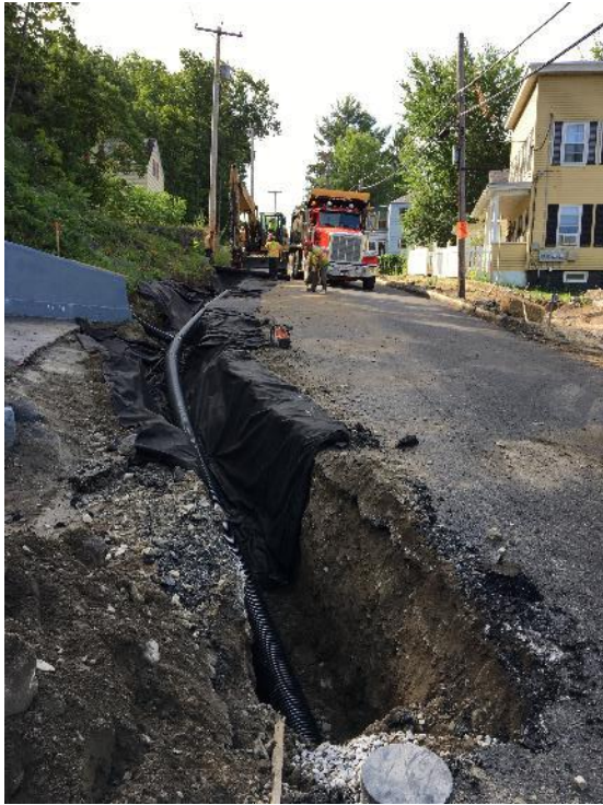
Figure 5 - Beech St underdrain
