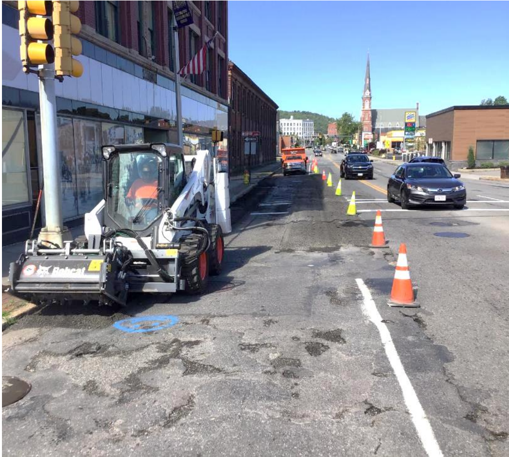
Figure 2 - Grinding Main Street
