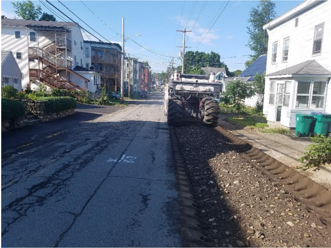
Figure 2 - Grinding up Beech Street
