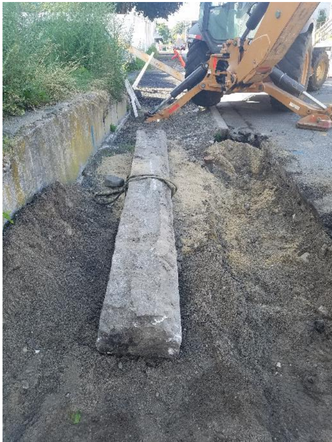
Figure 1 - Clarendon Curb Reset
