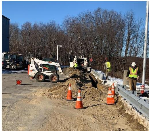
*Fig. 2: Gas Service Replacement Work (trenching along guardrail, at East WWTF).*
