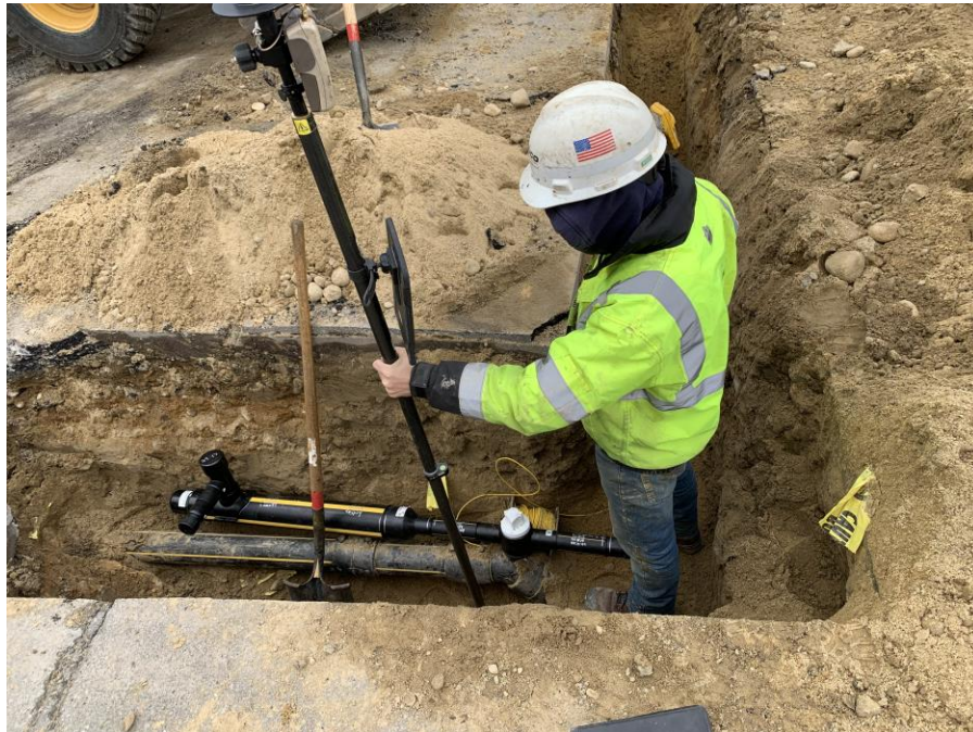
Figure 2 - Tie-in gas line project
