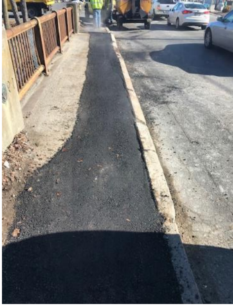
Figure 1- Lunenburg Street sidewalk repairs
