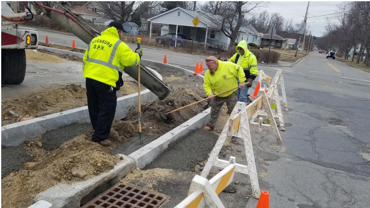
Figure 1 - DPW cementing curb
