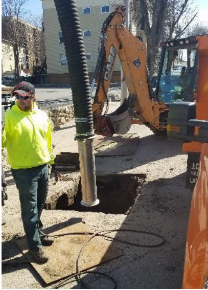
Figure 1 - Vacuum Excavation
