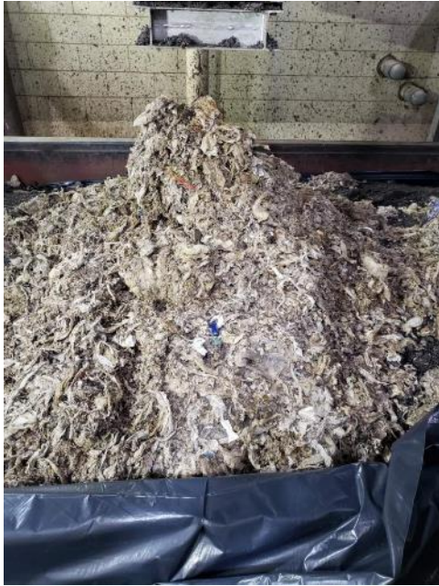
Figure 4 - Rag Blockage at WWTF
