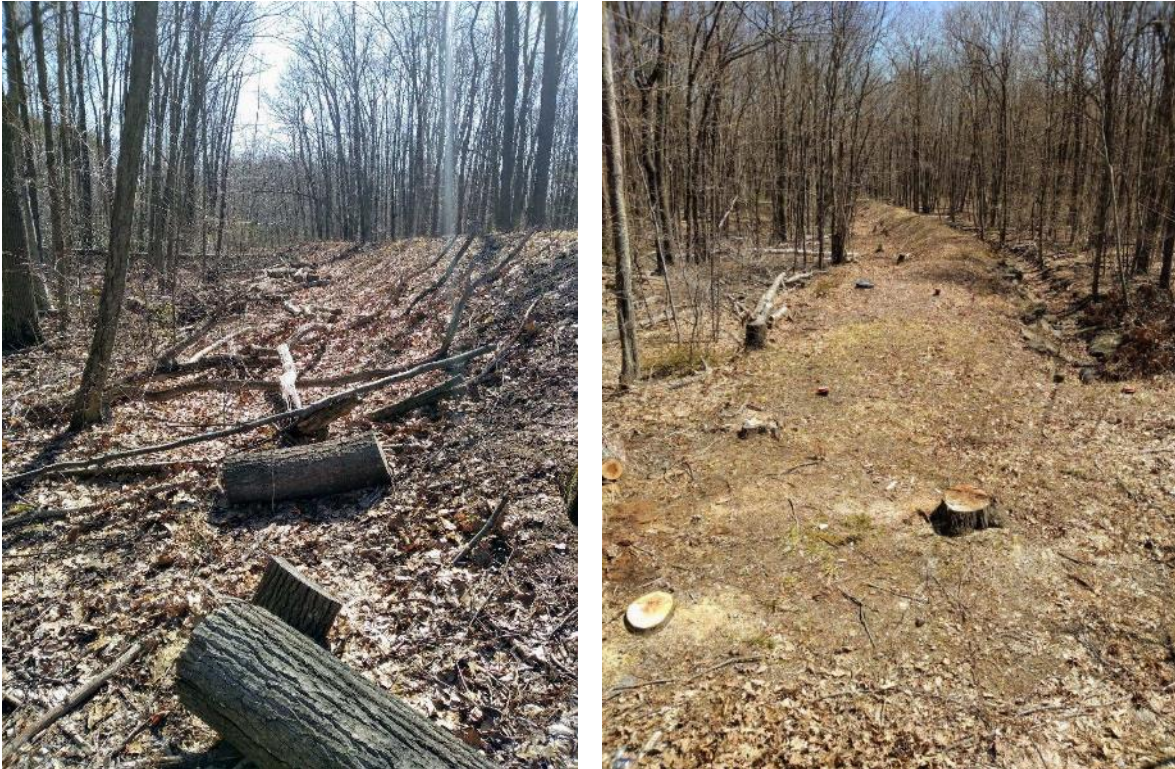
Figure 3 - Clearing of Transmission Main
