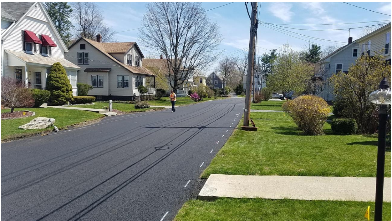
Figure 2- Laying out Berms on Berkley St
