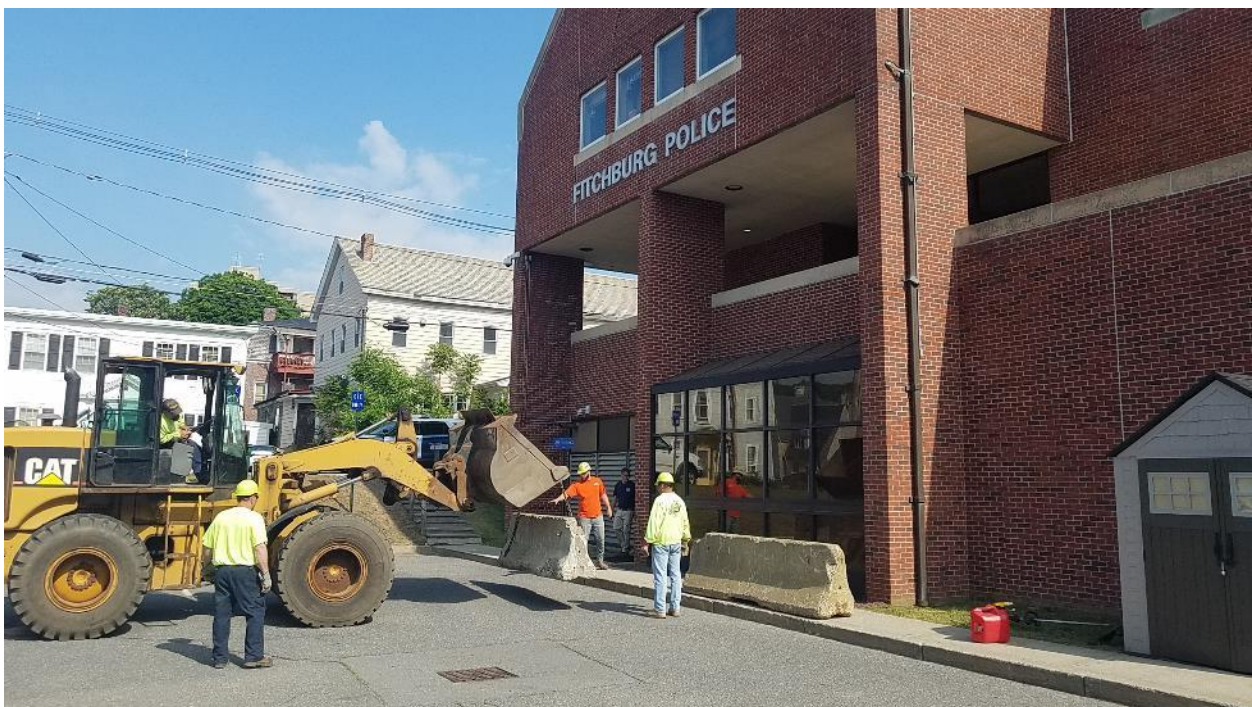
Figure 1 - Installing Barriers at FPD
