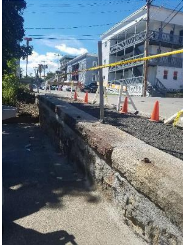
Figure 2 - Sidewalk repair Daniels at Pratt
