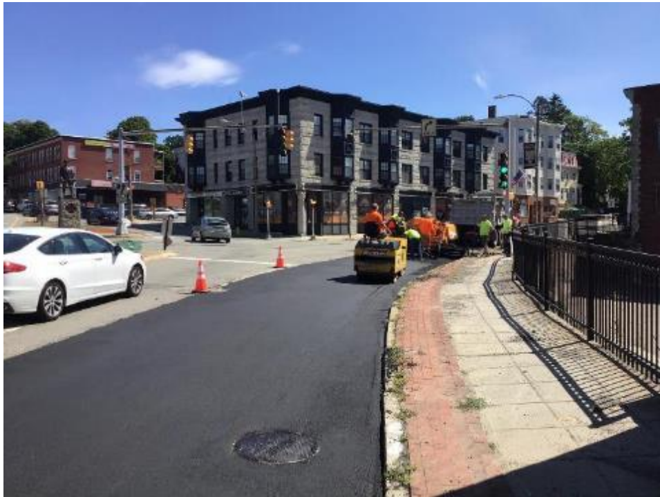
Figure 1 - Paving Moran Square
