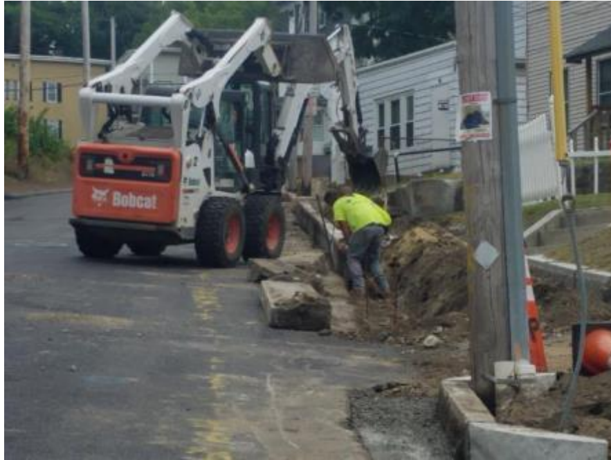
Figure 3 - Resetting Curb on lower Beech St
