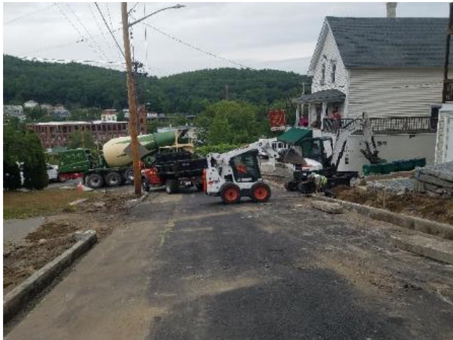
Figure 4 - Final section of curbing
