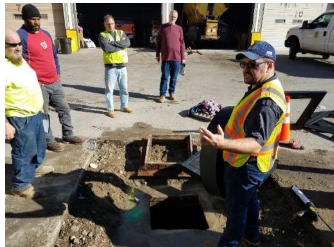
Figure 1: Cretex representative giving demo to Streets & Sewer personnel of PRO-RING™ riser rings in DPW Yard.
