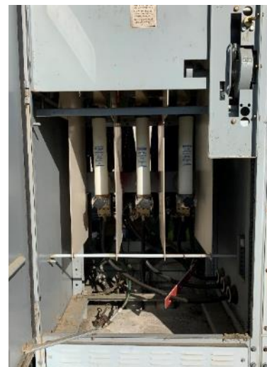
Figure 3: Replacement High Voltage, 100A Fuses.
