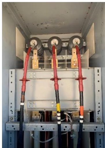
Figure 3: Replacement Transformer Feeders.
