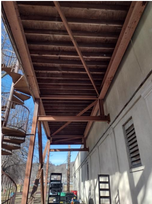
Structural Steel Frame (At Press Box Floor, paint steel bracing but not timber floor joists and flooring)
