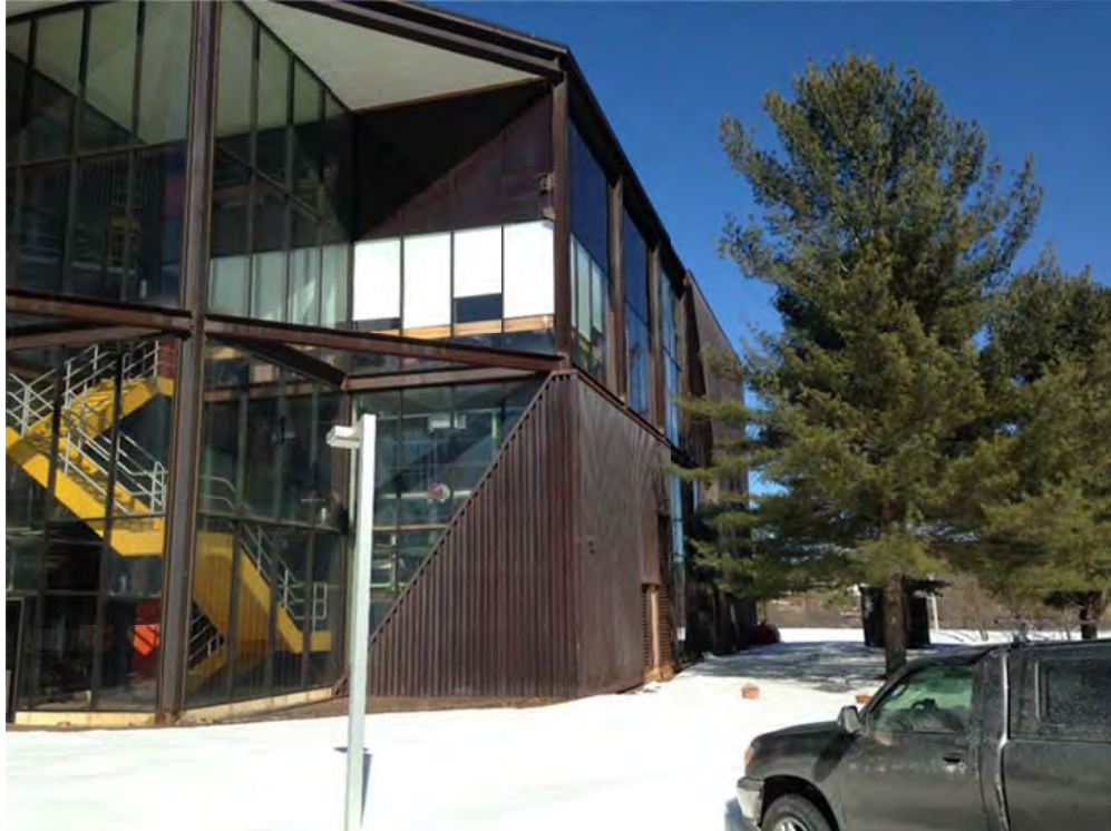
Photo 14: East entry of filter building, facing north 3/6/2014
