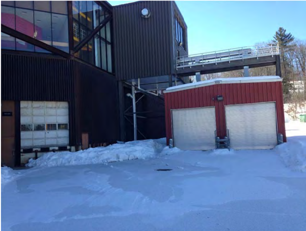
Photo 19: Filter building, facing north. Note existing conveyor and hopper garage 3/6/2014
