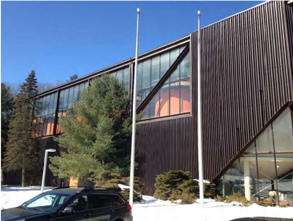
Photo 15: Front of filter building, facing northwest 3/6/2014
