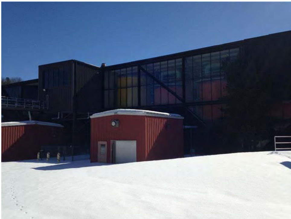
Photo 22: Rear of filter building, facing east-southeast
