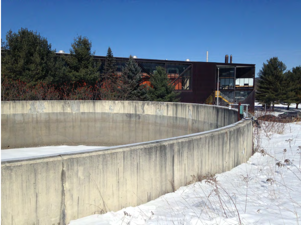
Photo 27: Existing backwash lagoon, facing north
