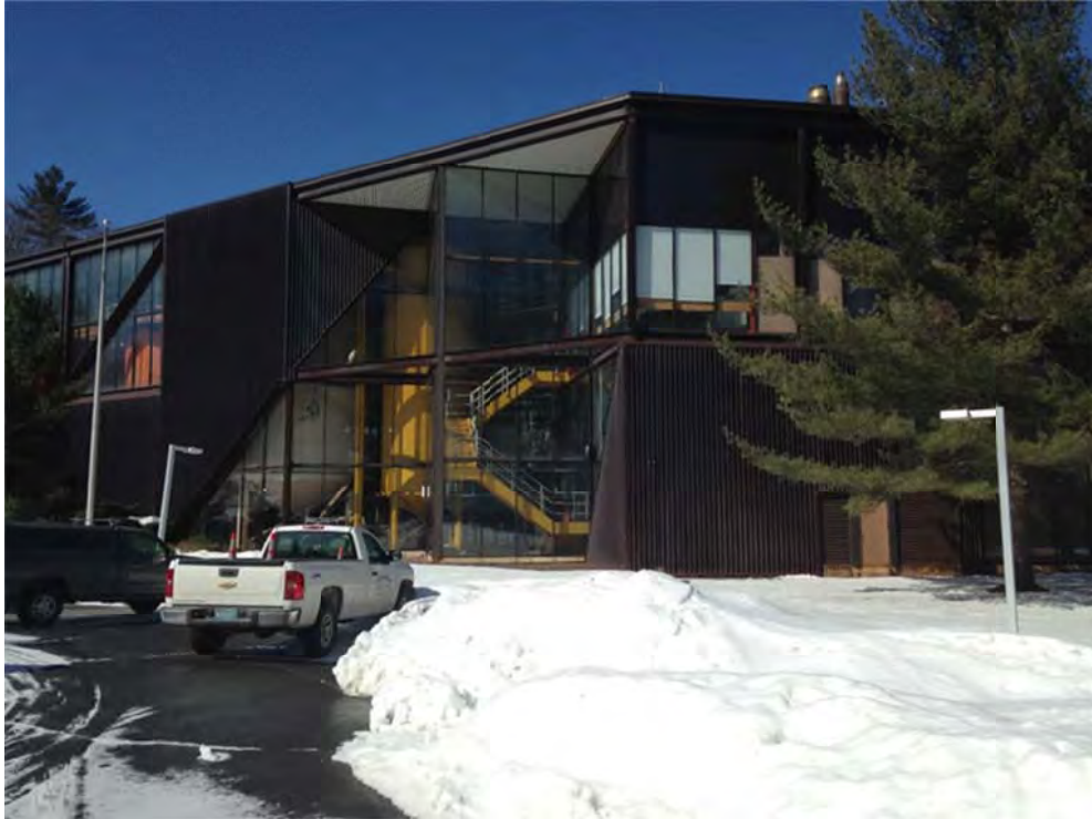
Photo 17: Filter building, facing northwest 3/6/2014
