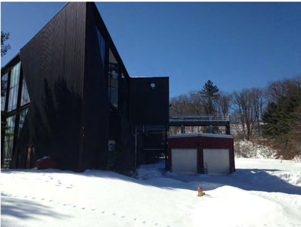
Photo 18: Filter building, facing northwest 3/6/2014
