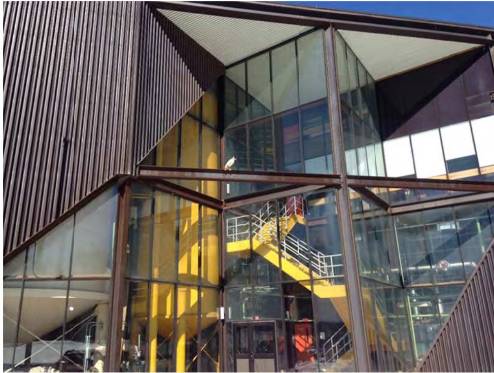
Photo 13: Filter building, facing west. Note transformer and 1,000 gallon AST 3/6/2014
