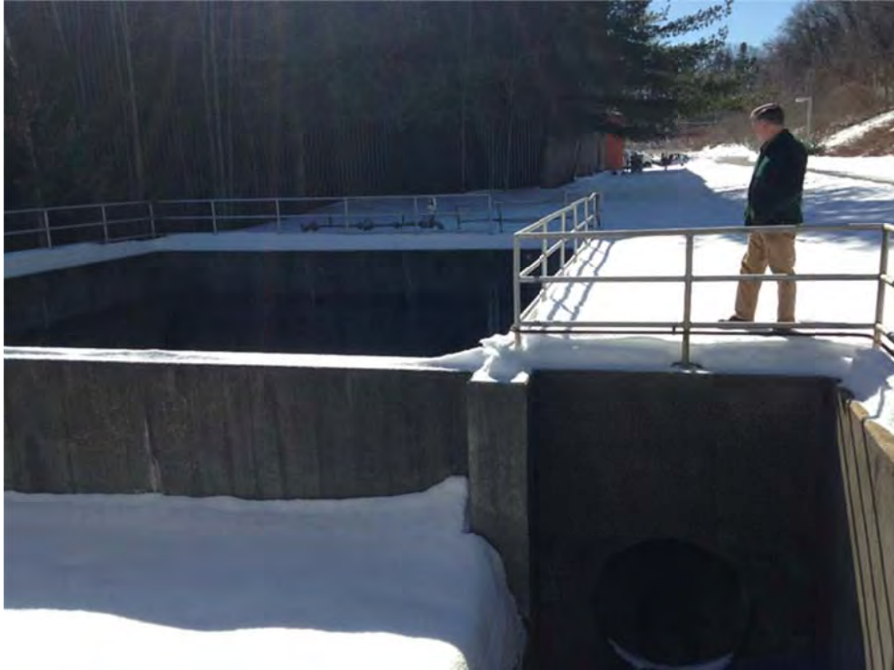
Photo 23: Post-aeration basin and effluent structure, facing south 3/6/2014
