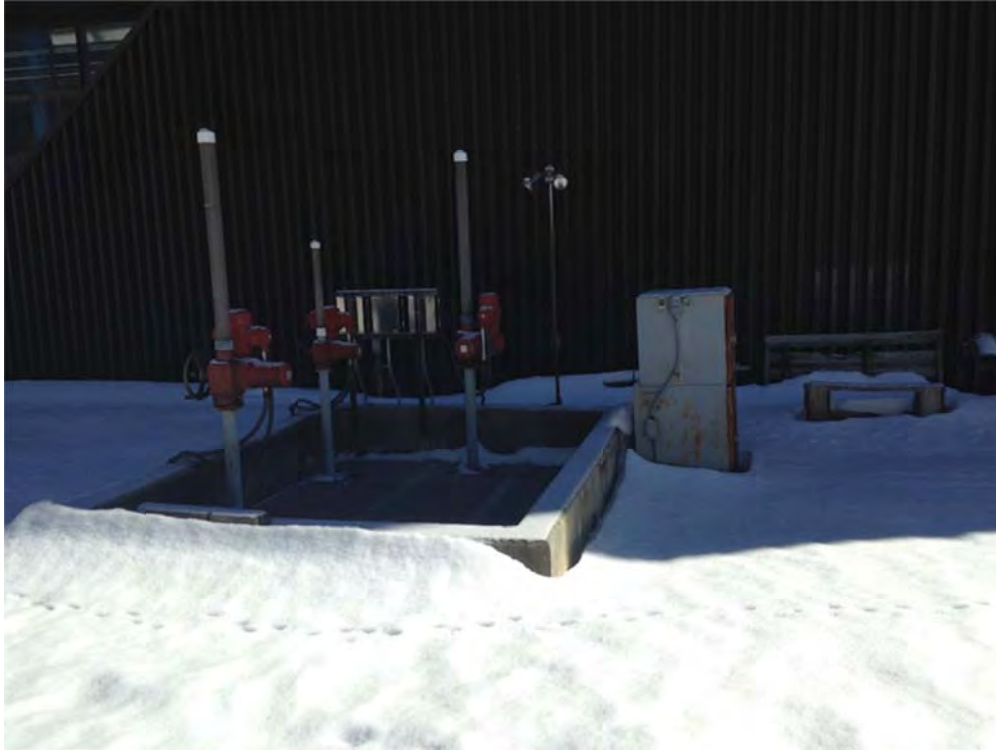
Photo 25: Filter bypass structure, facing east 3/6/2014
