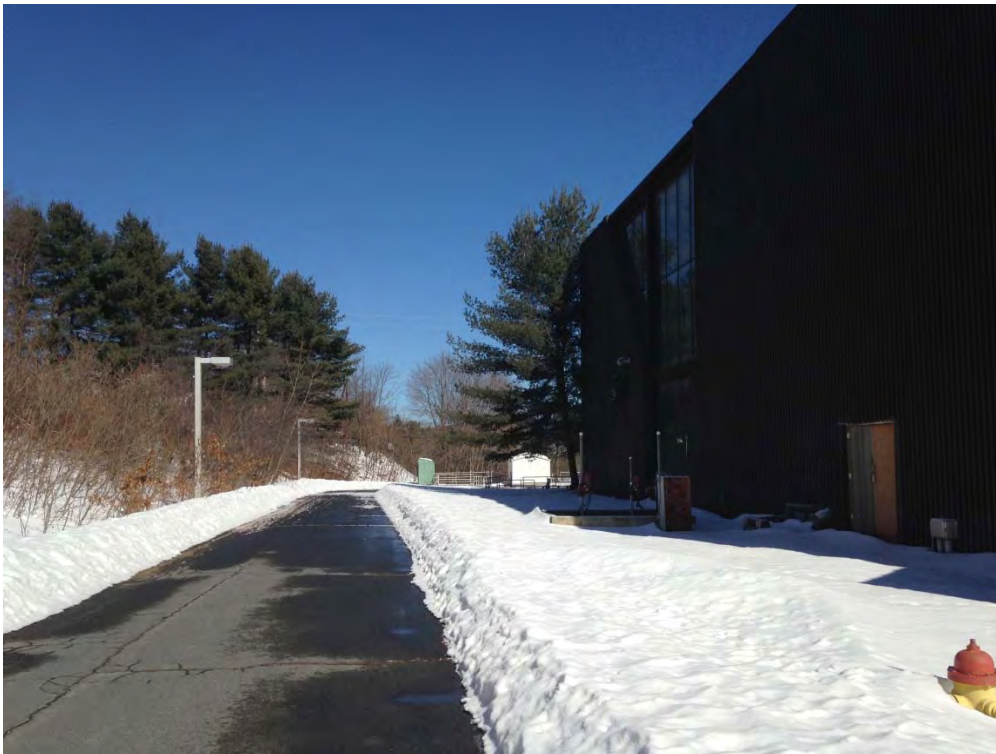
Photo 56: Existing Access Road, facing north 3/6/2014
