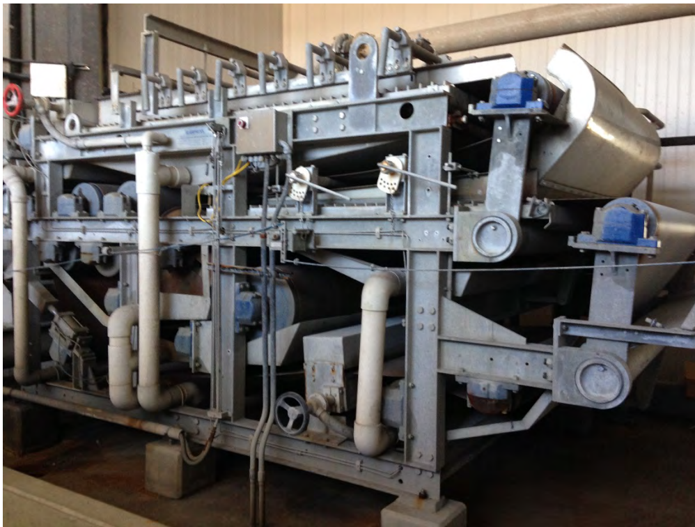
Photo 2: Klampress® belt filter press (2 of 2) 3/6/2014
